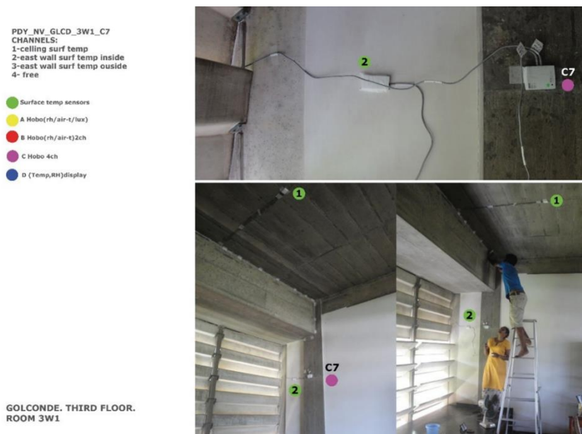
Figure 20 Placement of loggers on the Third Floor - Inside the room
