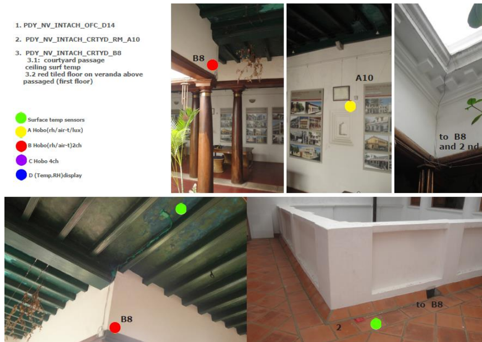
Figure 28 Placement of loggers in INTACH office – site photos
